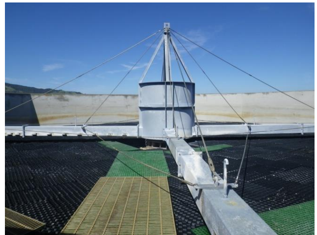
New rotary distributor, Biotower No. 2
