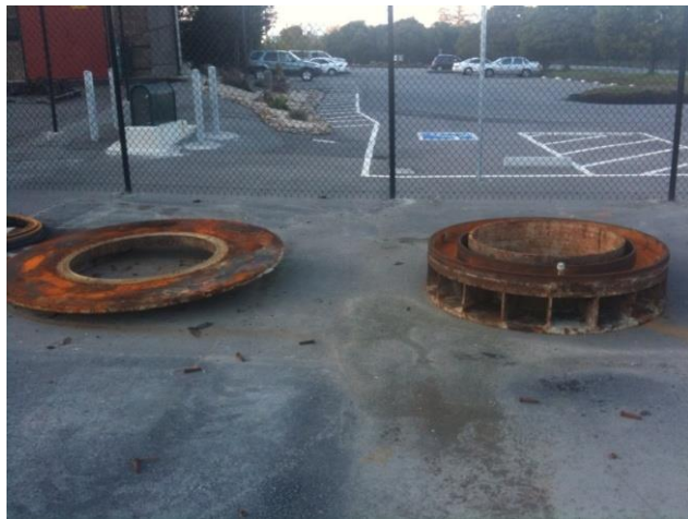
Original base & turntable, Biotower No. 2
