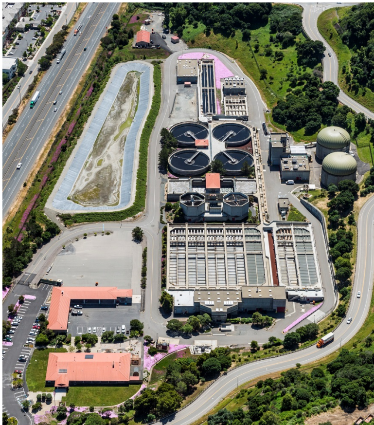
(Clockwise upper left to right): Effluent Storage Pond, Maintenance Annex (red roof behind the pond), Chlorination/Dechlorination Building, Chlorine Contact Tanks, Effluent Pump Station, Secondary Clarifiers, Solids Handling Building, Organic Waste Receiving Facility, Digesters and Digester Building, Aeration Tanks, Biotowers, Primary Clarifiers and Blending Channel, Grit Building, and Headworks. The two orange-roofed buildings in the lower left are the Maintenance Building (top) and the Administration Building (bottom).
