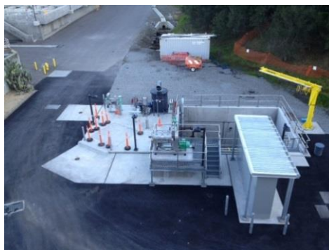
Organic Waste Receiving Facility
