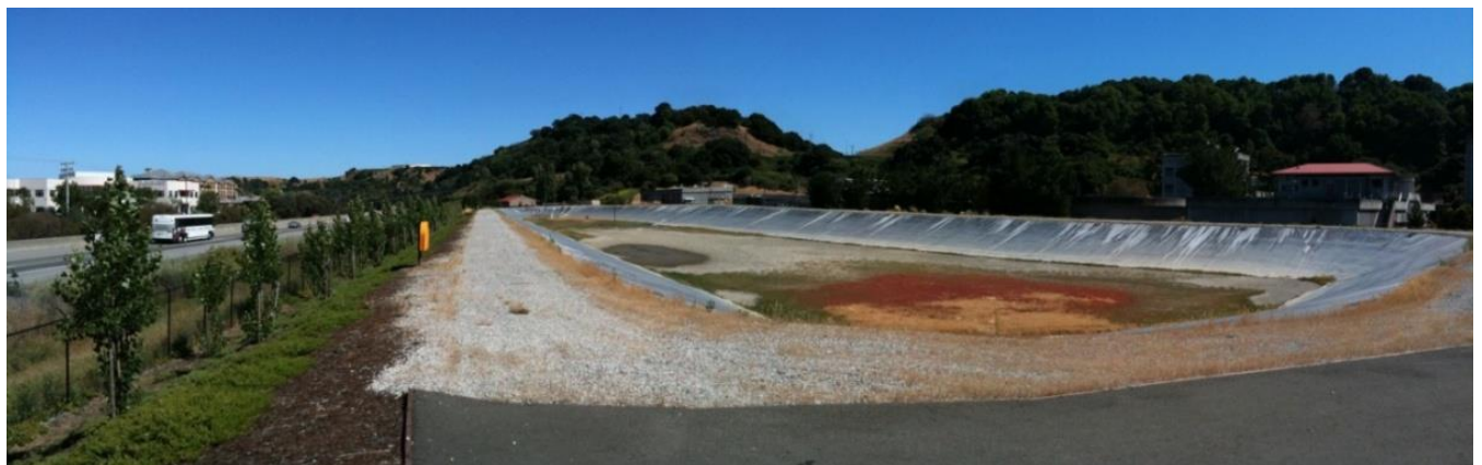
Effluent Storage Pond
