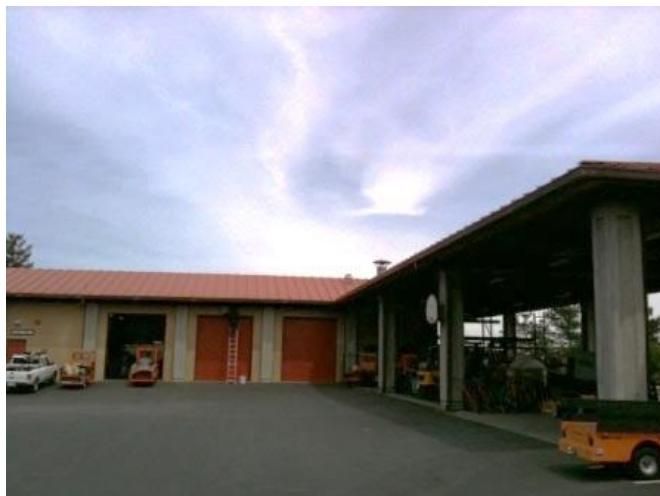
Maintenance Building and Covered Portico
