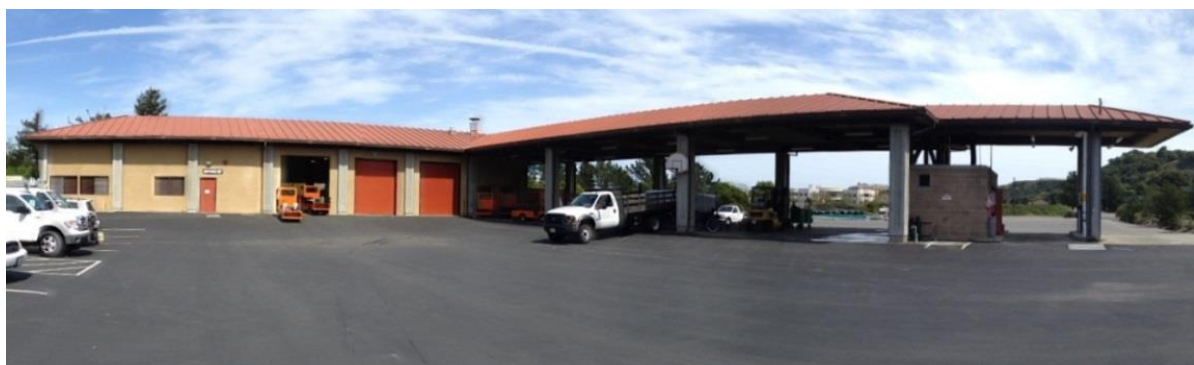
Maintenance Building with standing seam metal roofs.
